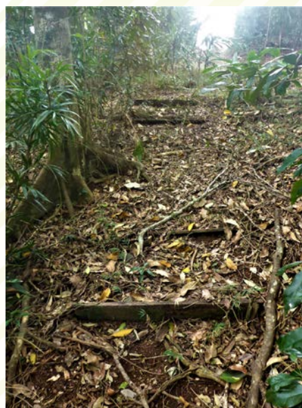
Historical steps forming part of a walking track built by WWII soldiers
