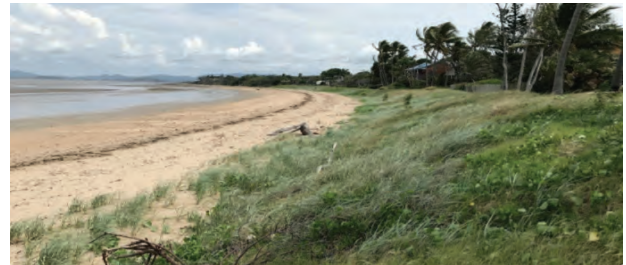
Buried geo-bag seawall at Zilzie, QLD
