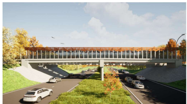
Figure 1 Artist impression of the new pedestrian and cyclist bridge west of the existing Stringybark Road bridge.
