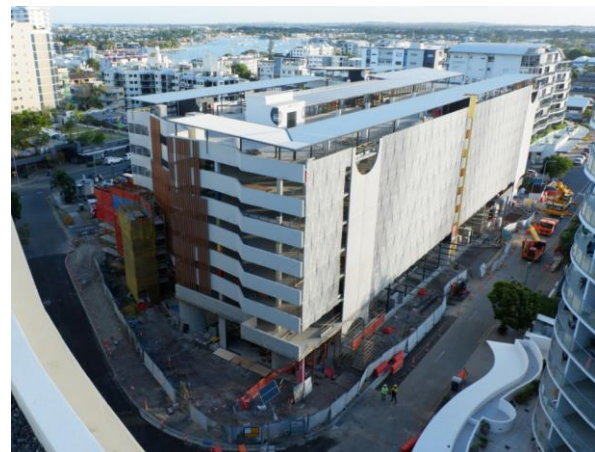
Mooloolaba new eight-storey car park
